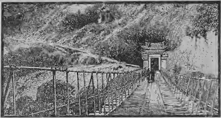
END VIEW, BRIDGE OVER PEPAN KIANG
